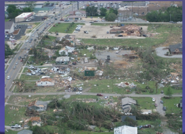
Up to EF-3 damage just S of Trenton
